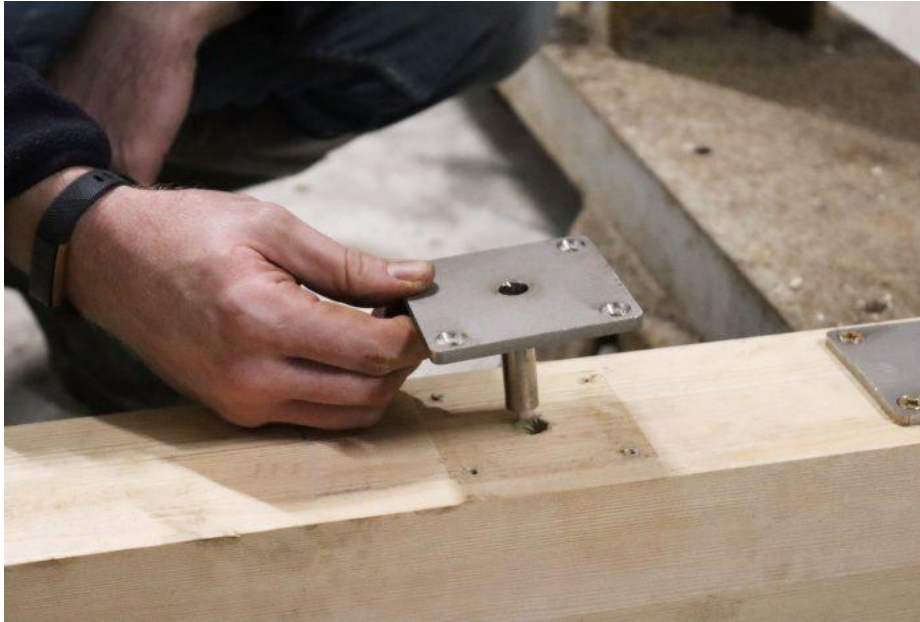
Plate 3 – Timber Fixing Plates
