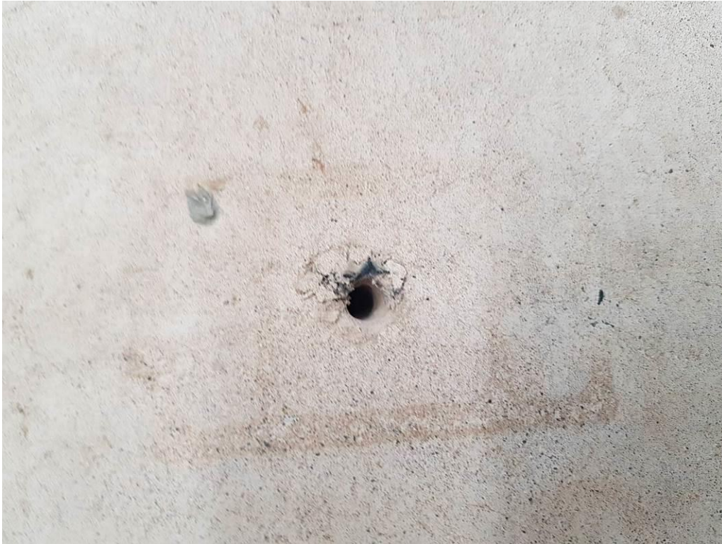
Plate 9 – Concrete Slab after Deconstruction
