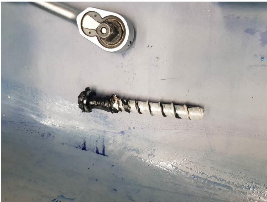
Plate 6 – Concrete Bolt used to Anchor Balustrade System
